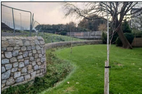
Existing Overland flow channel at Clon Brugh
