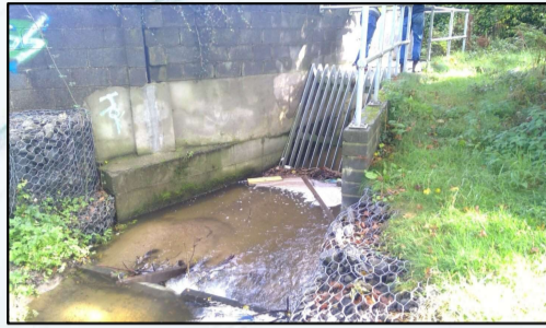
Existing Inlet structure at Belarmine Park
