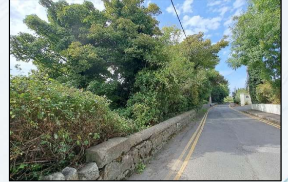
Existing wall to be replaced at Ballyogan Grove
