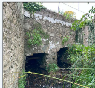
Kilgobbin Road Bridge
