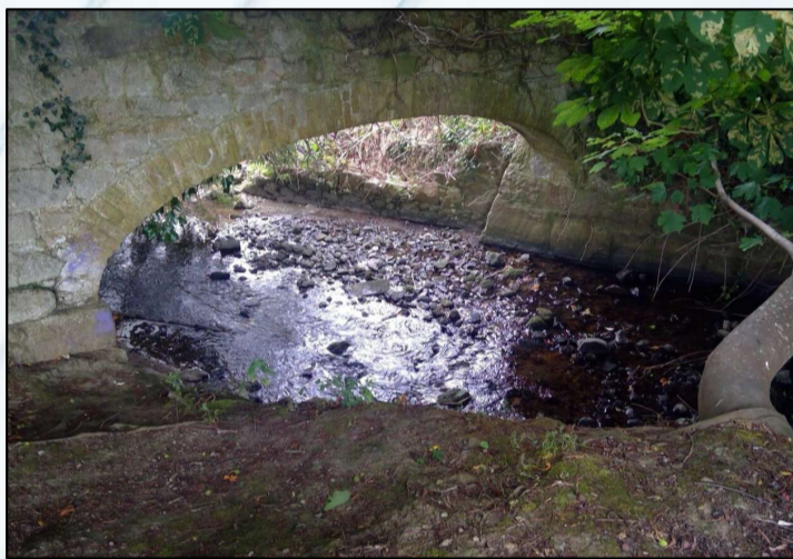
Existing masonry arch upstream of the works
