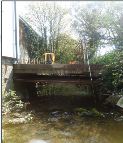
Existing footbridge across the works area
