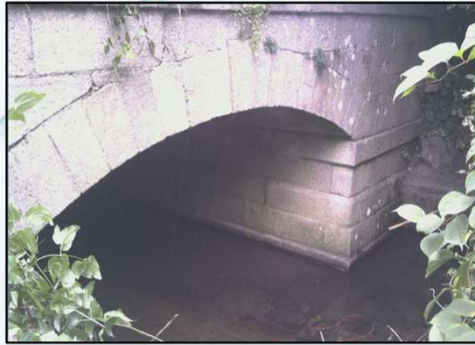
Existing N11 Culvert (Upstream)
