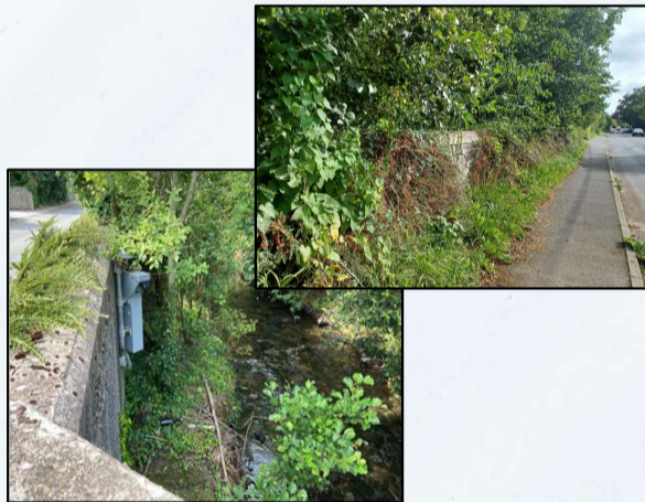
Existing flood defence walls at Commons Road
