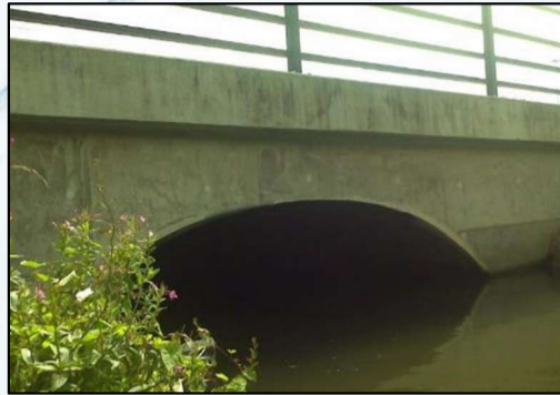
Existing culvert traversing Glenamuck Road North
