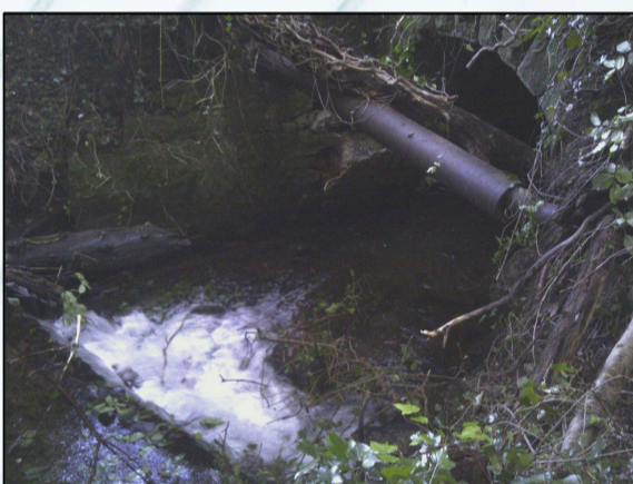
Existing inlet at Cherrywood Viaduct
