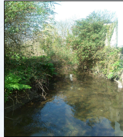
Channel widening section
