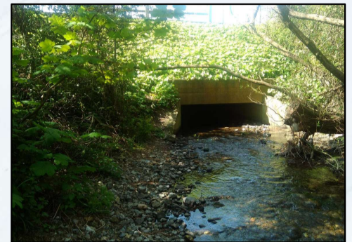
Existing N11 Culvert (Downstream)
